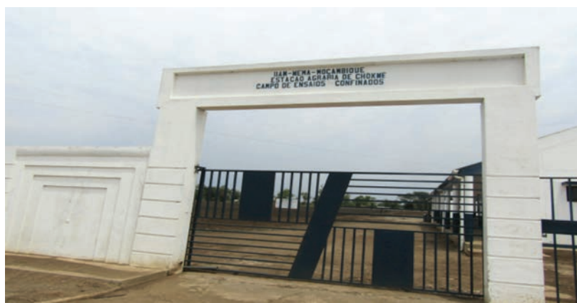
The WEMA infrastructure that will host the trials of GMO Maize in Chókwè
